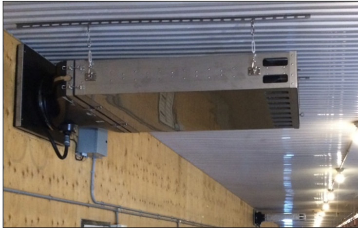
Figure 4 Typical installation of a counter-flow air-to-air HX unit in a broiler house
